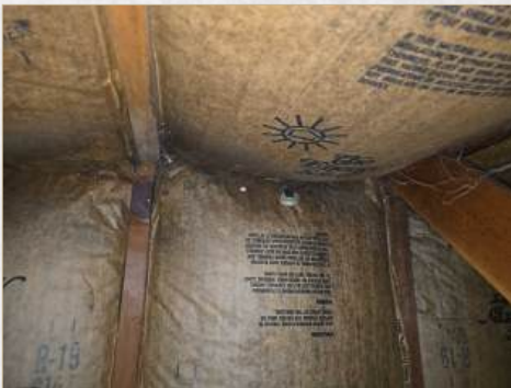
Evidence of past/present moisture entering, dry at time of the inspection, *see the roof section for conditions and repair or replace recommendations
