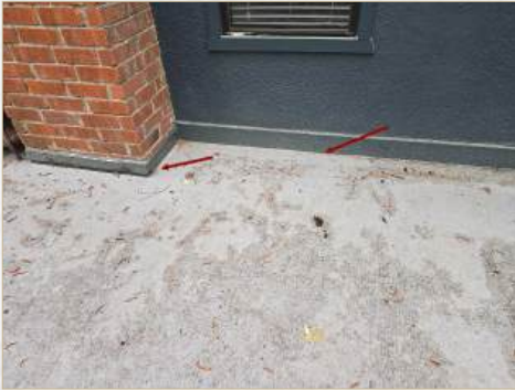
Flashing encapsulated at upper balcony deck, recommend further evaluation
