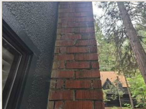
Improper grout tooling and loose grout present at chimney, recommend repair or replace
