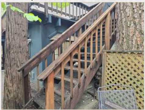
Handrail/guardrail openings too wide, normal for age of the structure, 4-3/8" maximum recommended for increased safety
