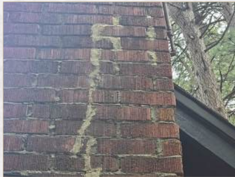
Improper grout tooling and loose grout present at chimney, recommend repair or replace
