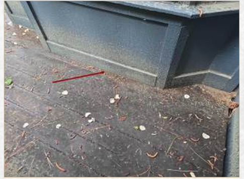
Missing wall to balcony flashing, recommend repair or replace | North side of structure
