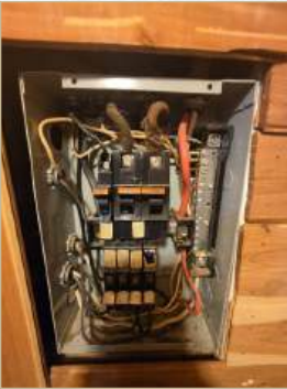
Zinsco/Sylvania/Federal Pacific/Stab-Lok electrical panel present, known to be problematic, recommend further evaluation
