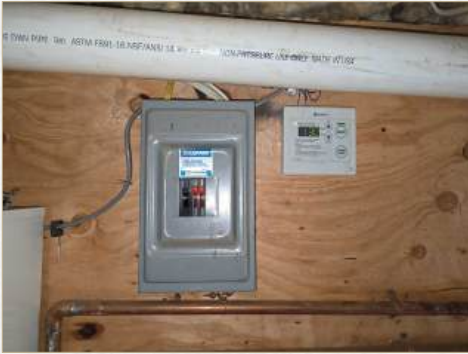
Zinsco/Sylvania/Federal Pacific/Stab-Lok electrical panel present, known to be problematic, recommend further evaluation
