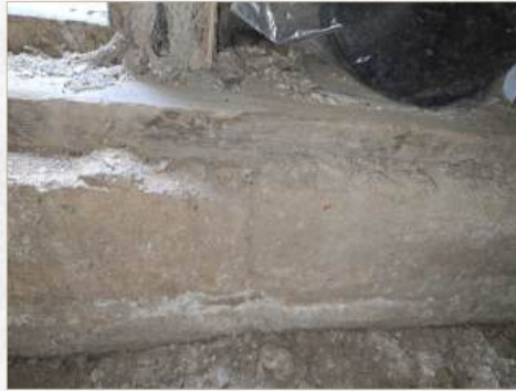
Minor cracks (less than 1/8-inch), typical for age and material
