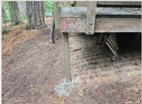
Trees affecting balcony, posts not plum or true, recommed further evaluation
