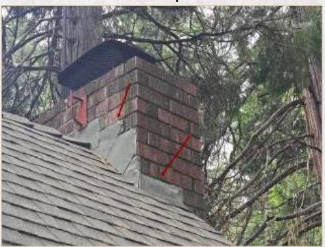
Flashing/mastic at base of chimney worn/loose/cracked, recommend maintenance to ensure a continued waterproof seal
