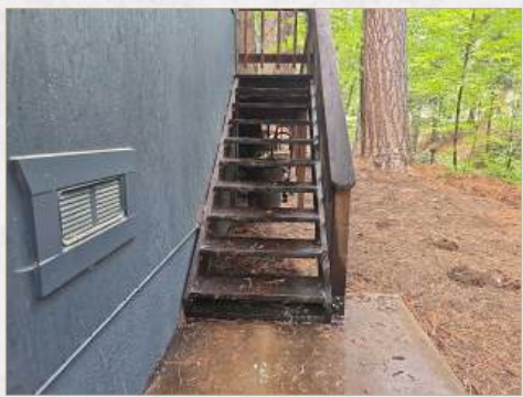
Open stair risers, potential safety issue for children, recommend repair or replace
