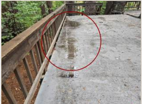
Ponding water/evidence of ponding, deck not draining properly, recommend further evaluation
