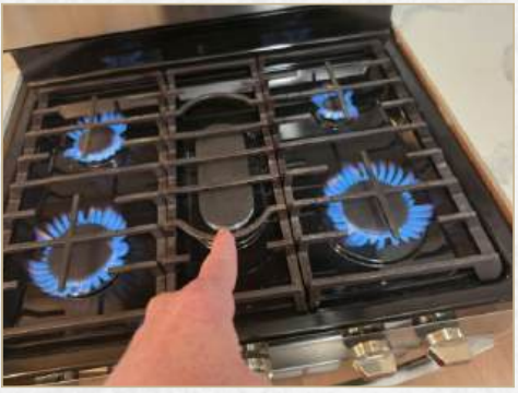
Center element/burner not operating, recommend repair or replace
