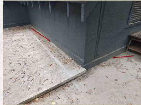
Missing wall to balcony flashing, recommend repair or replace | North side of structure
